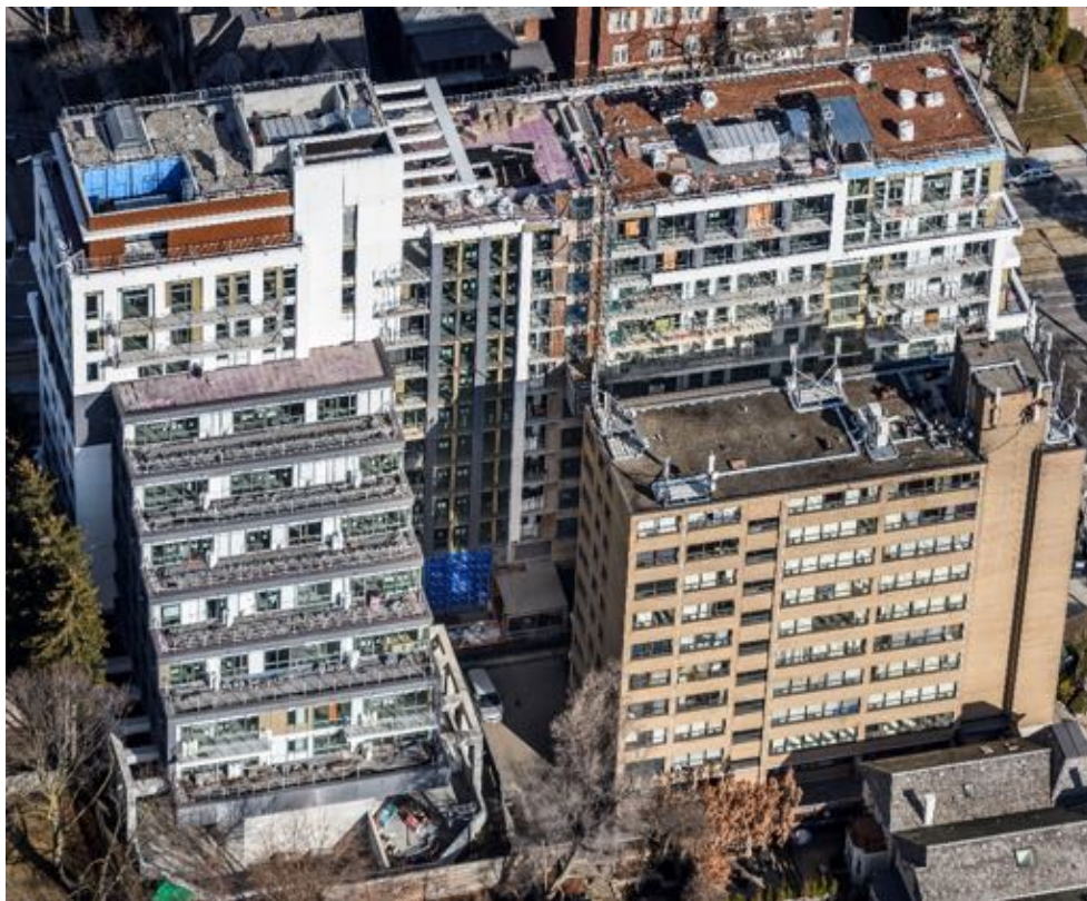
SOUTH ELEVATION MARCH 2018
